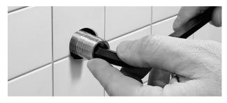
4. Tighten the extender into the Lugged elbow with the provided Allen Key.
