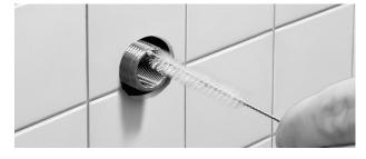
2. Use the brush to remove all loose brass from inside the lugged elbow.
