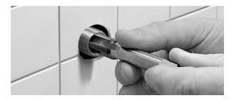
Using the provided tap, cut a thread inside the lugged elbow. Taking care to make the thread straight.
